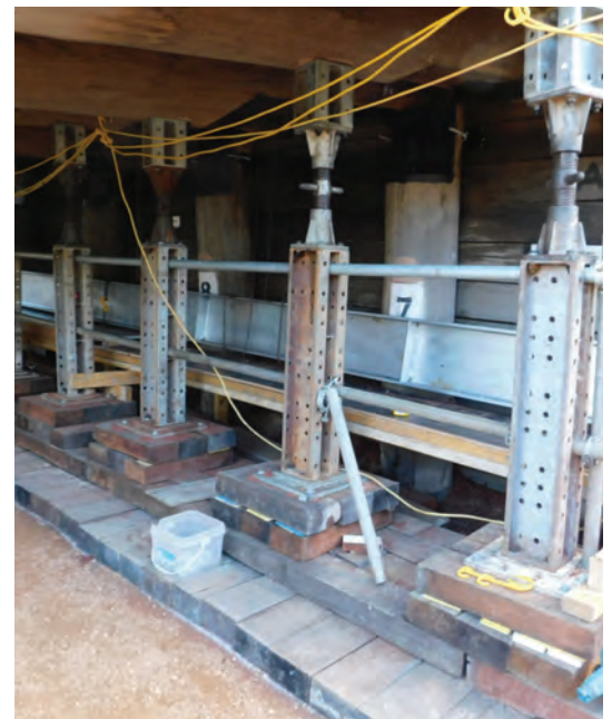
50T props supporting bridge stringers during strengthening work.
