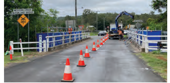
Overview of McFarland bridge with traffic management.
