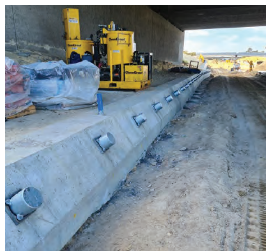
Capped and completed ground anchors.
