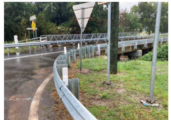
New bridge guardrail installation.
