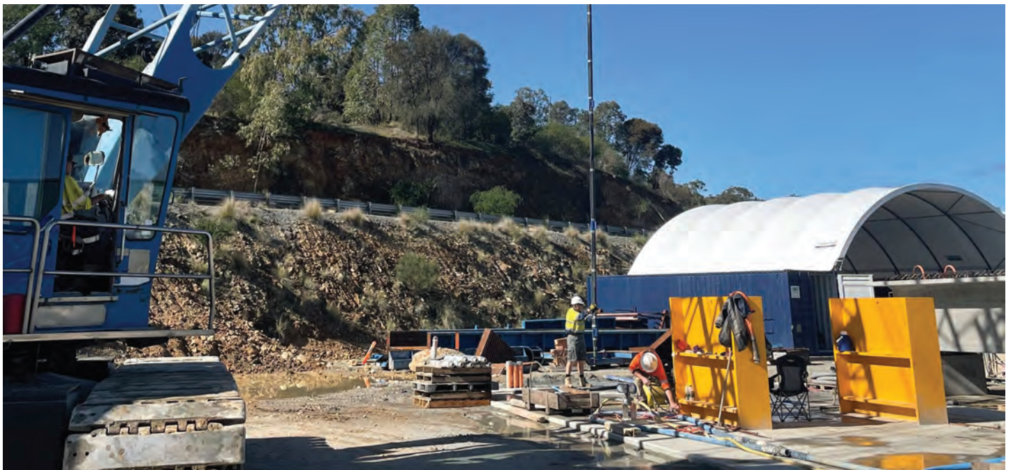
Ground anchor installation by crane.
