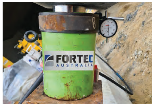
Load testing with movement monitoring.
