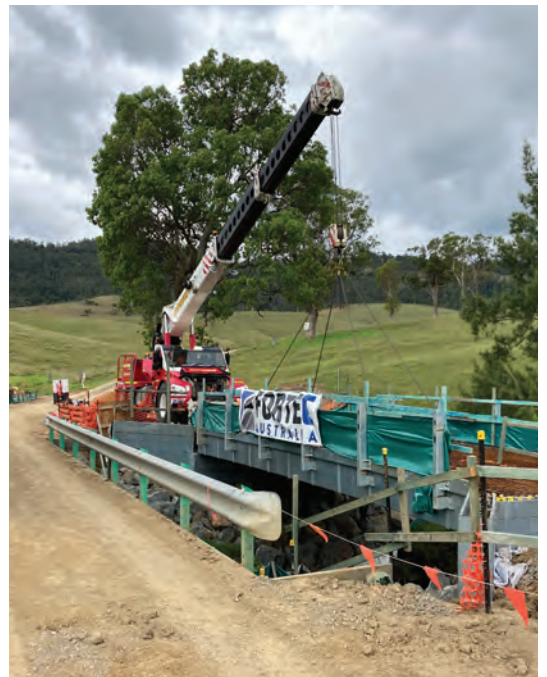
Earthworks starting for the construction of the first bridge.
