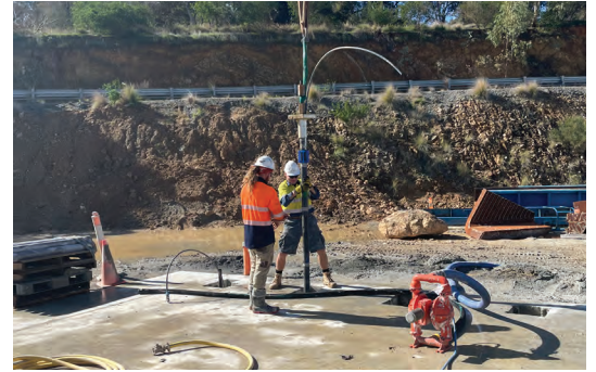
Installation of the DCP anchor.
