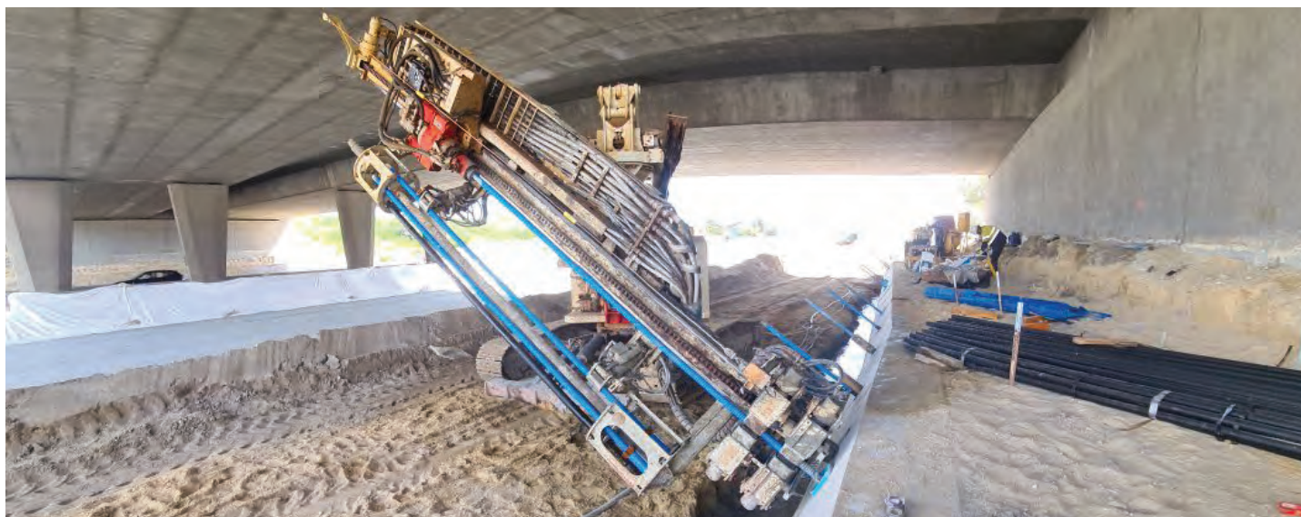
Drilling for ground anchors under existing bridge.
