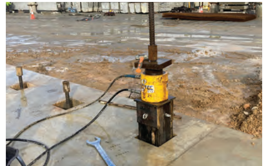
Load testing and stressing.
